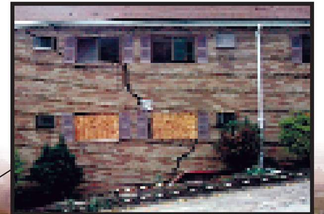
Illustration of Trough Subsidence.
