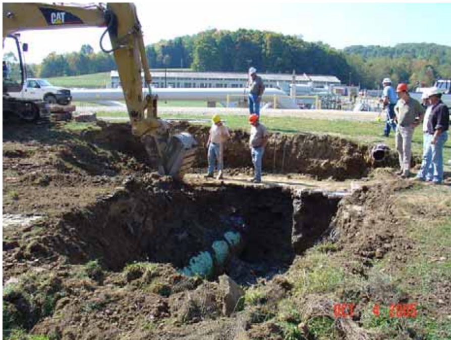
Photo IV-13f: DEP Photograph taken on October 4, 2005 showing a Texas Eastern pipeline being exposed for repairs.
