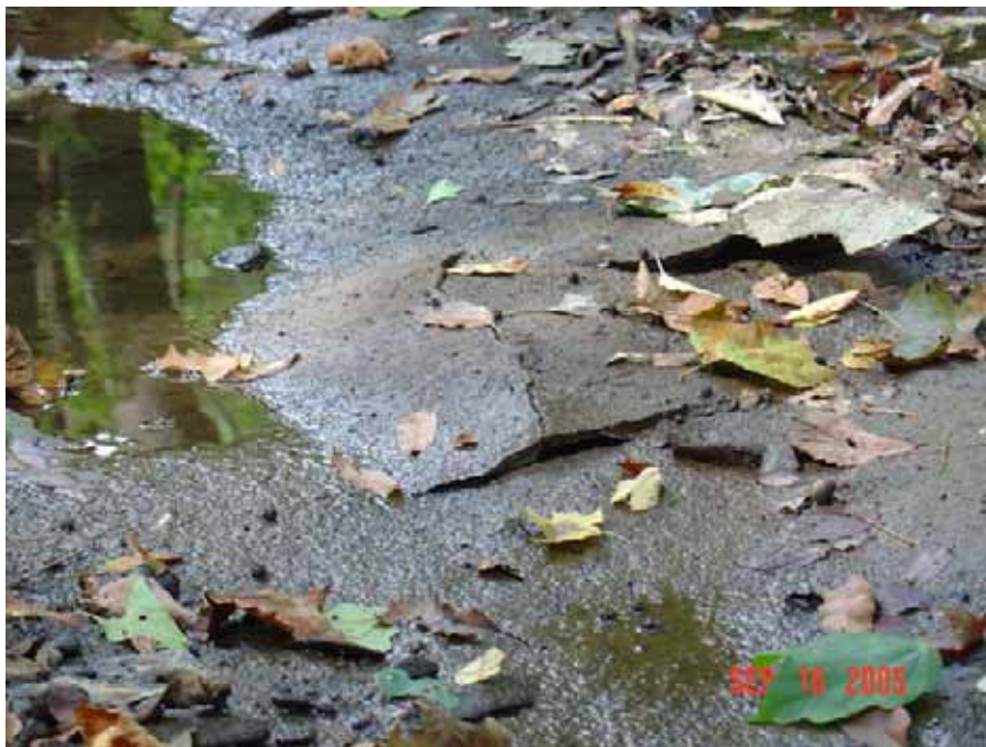
Photo IV-11d: DEP Photograph taken September 16, 2005 showing heaved and cracked rocks within streambed.
