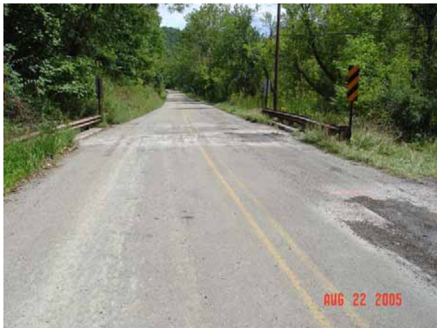
Photo IV-2a: DEP Photograph taken on August 22, 2005 showing view of Bristoria Road Bridge from the northwest.
