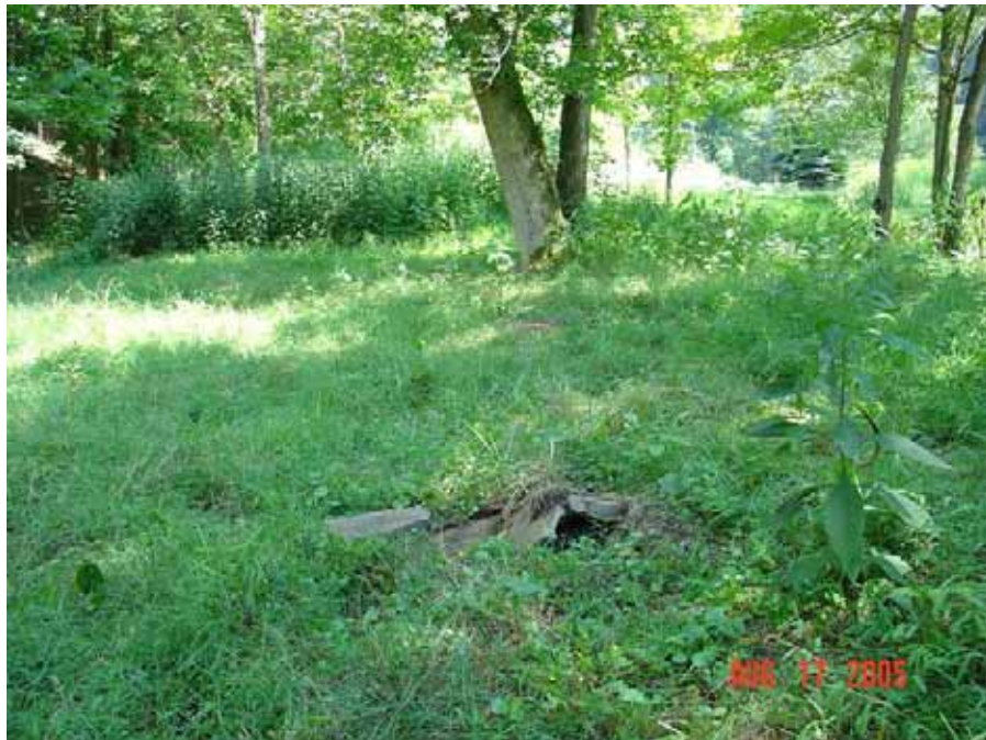
Photo IV-4b: DEP Photograph taken on August 17, 2005 showing ground heave with gas line heave in background.
