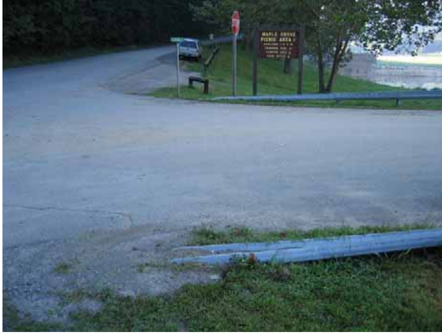
Photo IV-5a: DEP Photograph taken on September 8, 2005 showing guide rail moorings on eastern end of Lazear Lane Bridge.
