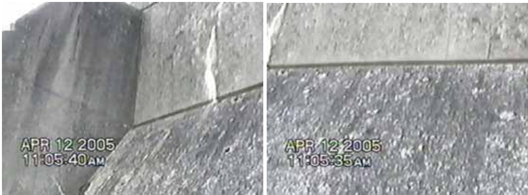
Photo II-15 and II-16 : CPCC video, taken April 12, 2005, shows little to no damage in this area at this time.
