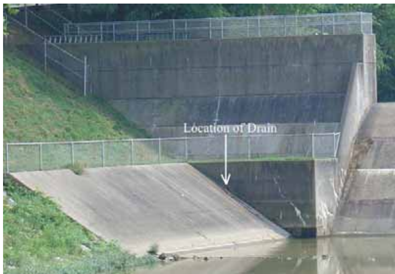
Photo II-10 : DEP photograph showing the location of the drain being referenced in this section.
