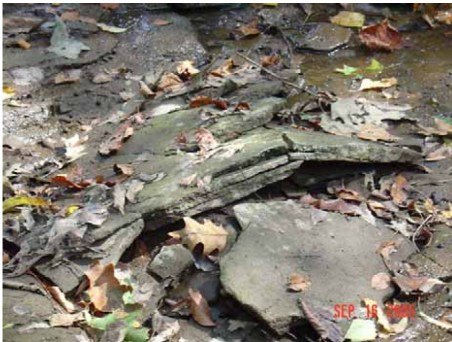
Photo IV-11b: DEP Photograph taken on September 16, 2005 showing heaved and cracked rocks within streambed.
