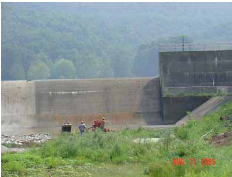
Photo II-6 : DEP photograph, dated August 11, 2005, shows a view of Ryerson Station Dam spillway and the left (west) side.
