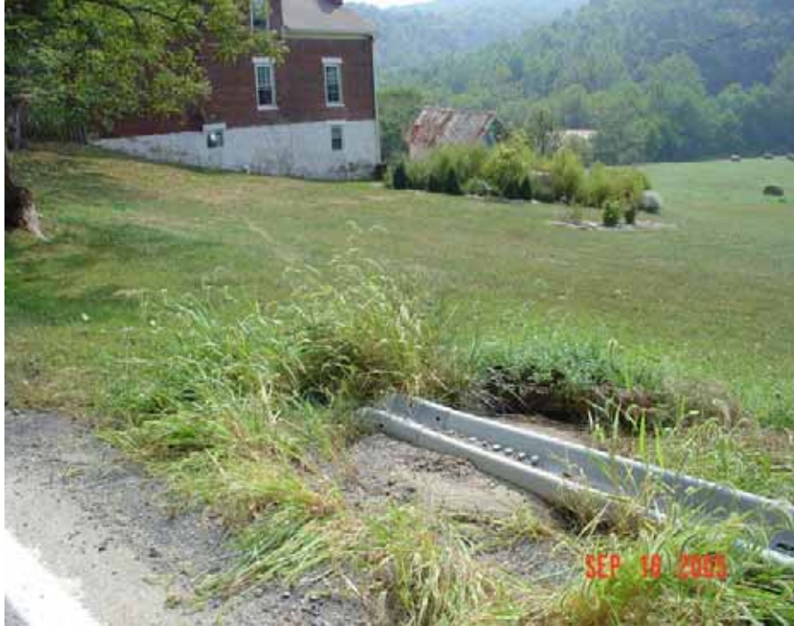
Photo IV-10a: DEP Photograph taken on September 16, 2005 showing southeastern guide rail mooring.
