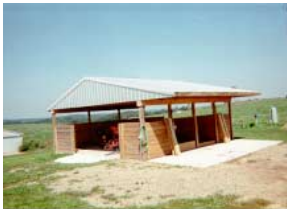
Figure 4. Four Bin Arrangement For Poultry Mortality. Bins are for primary (2), secondary and amendment storage. Additional space is for storage of material prior to land application.
