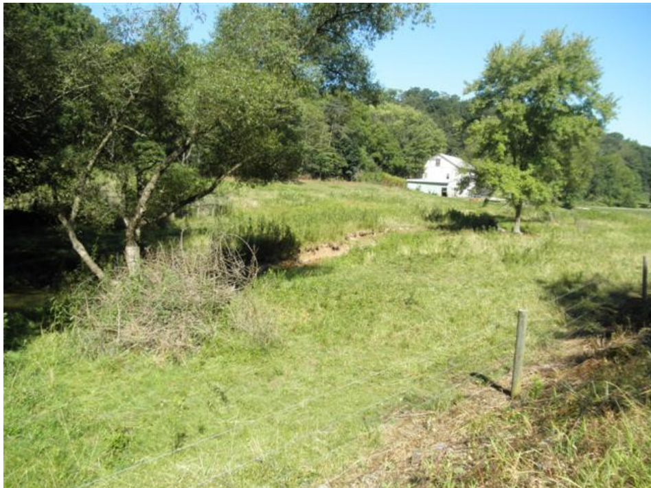
Figure 4. Stream bank erosion in the Hoffer Creek Watershed.
