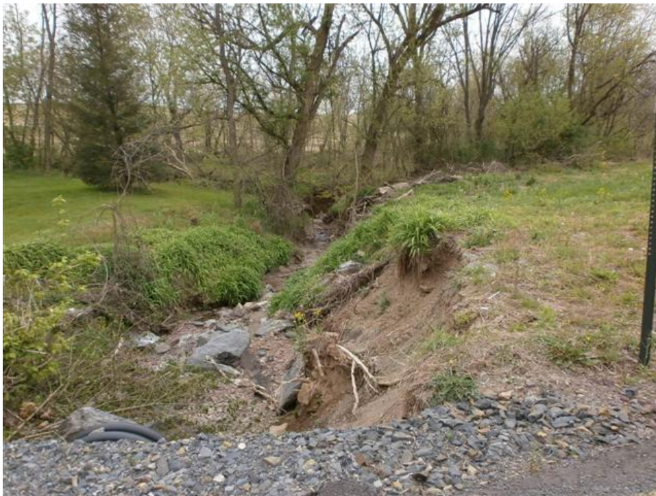
Figure 4. Stream bank erosion in the Montour Run Watershed
