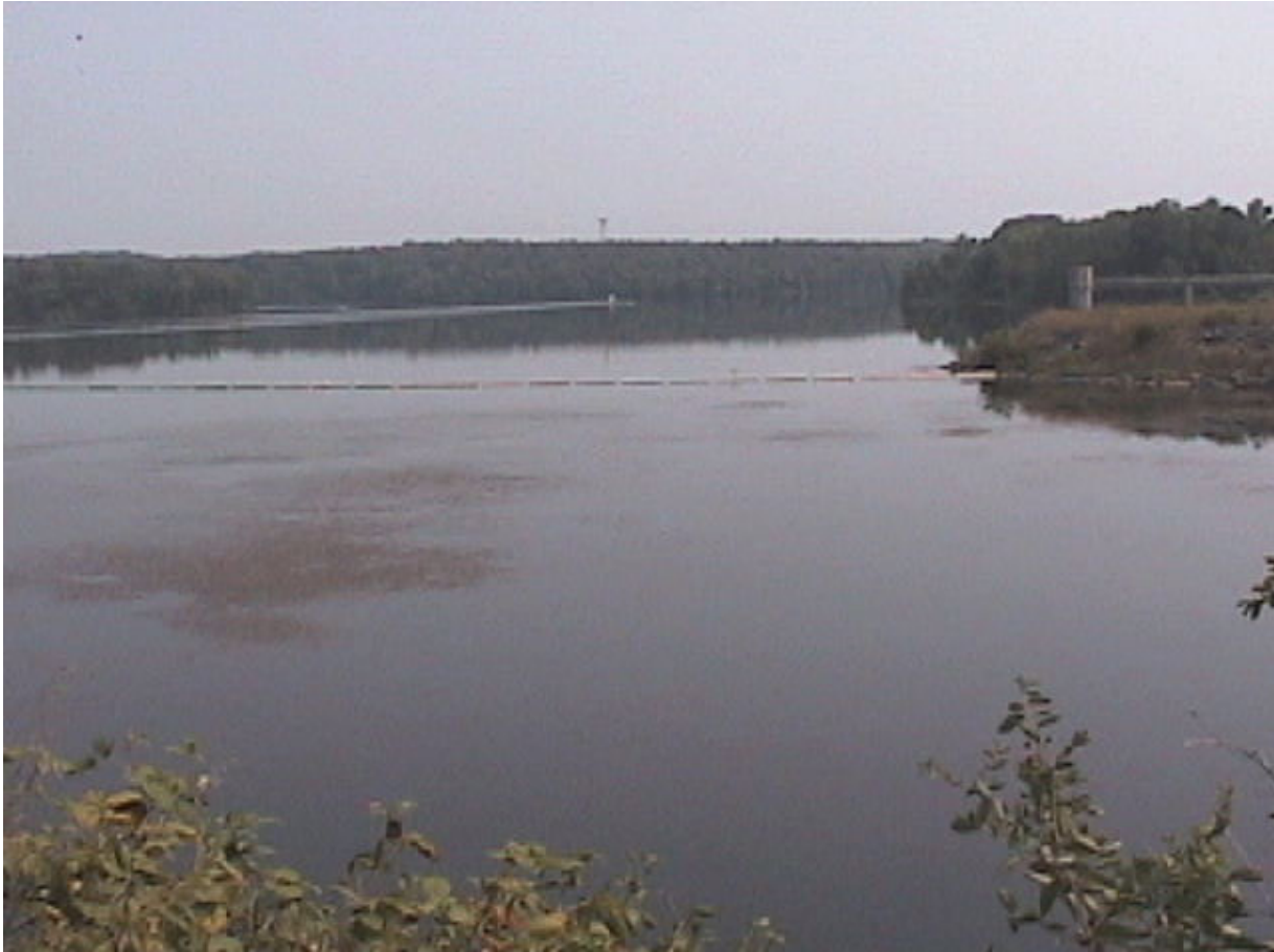
Picture 1-1. View of Lake Nockamixon from the dam.
