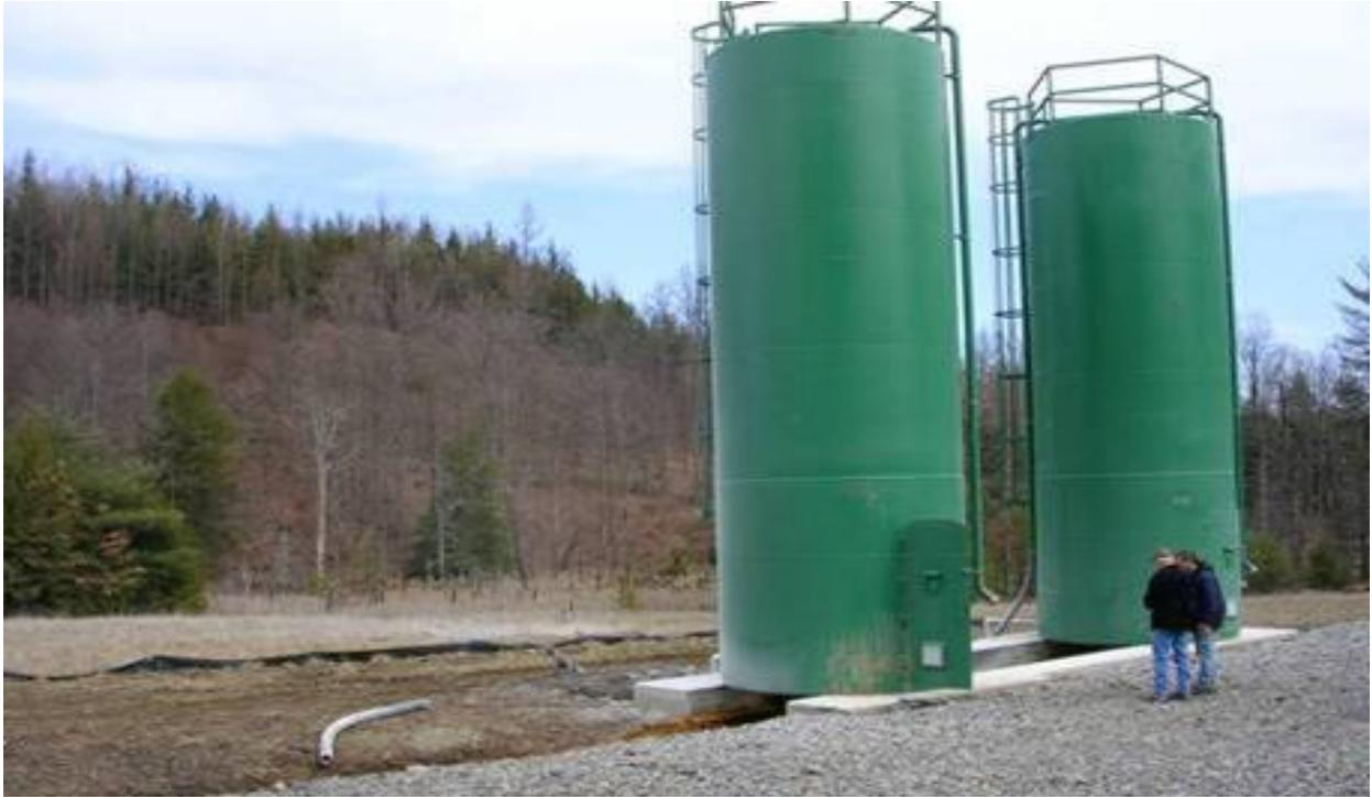
Figure 20. Lime silos for a tipping bucket lime doser treating another mine discharge in the Porcupine Hollow Tributary of Dents Run.
