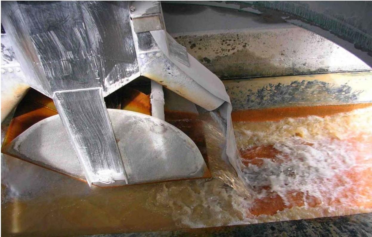
Figure 21. Tipping bucket mechanism dispensing lime to neutralize the highly acidic discharge.
