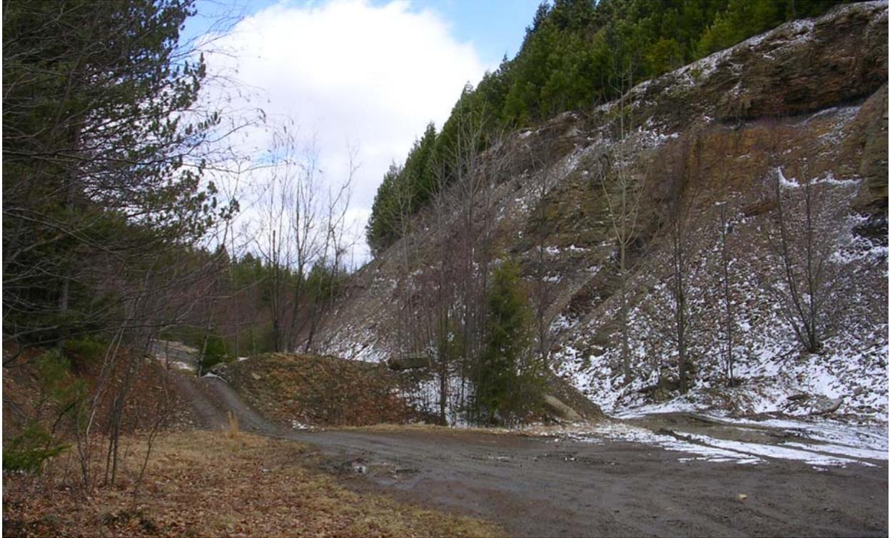
Figure 15. High-priority unreclaimed dangerous highwall located on State Game Lands in the Bennett Branch Watershed.
