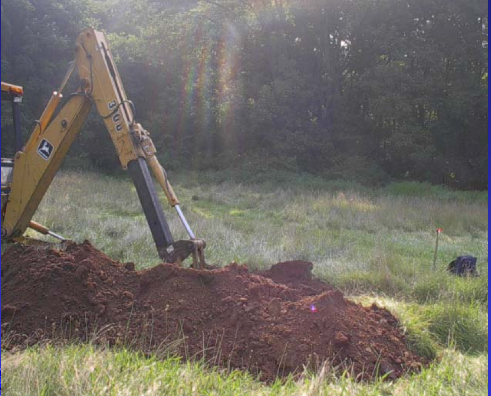
Excavation of deep hole by backhoe
