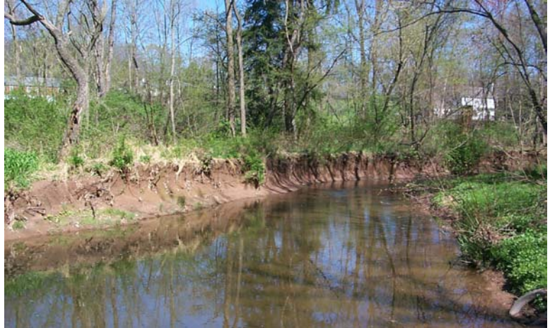
Undercut streambanks are a common impact of increased stormwater runoff.
