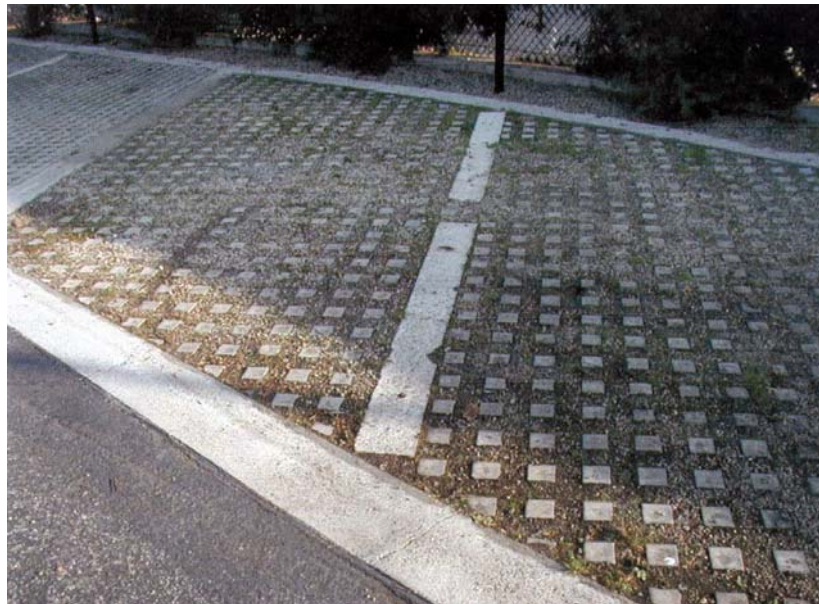
Figure 5.10-2. Overflow parking using permeable pavers
