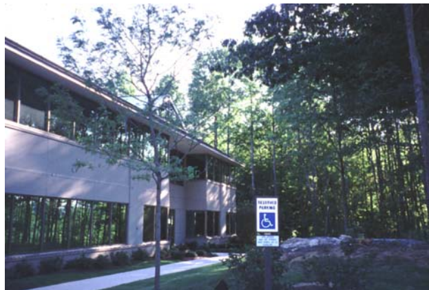
Figure 5.6-3 Woodlands Protected through Minimum Disturbance Practices
