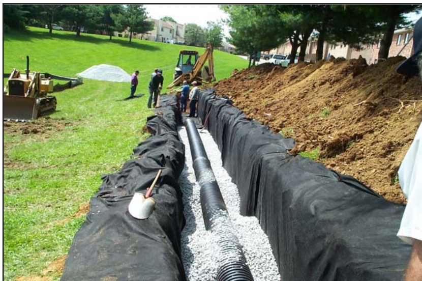
Figure 6.4-5. Installation of Infiltration Trench
