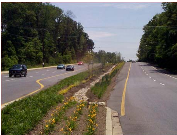
Figure 6.5-10. Example of rain garden treating highway runoff (LIDC)
