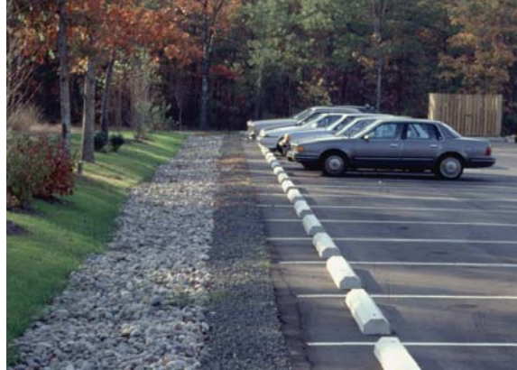
Figure 6.1-22 Porous parking lot w/ stone edge drain at the SmithKline Beecham Site
