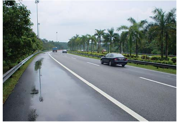
Figure 6.1-20 Porous asphalt highway (standard asphalt shoulder) in Japan, courtesy of Infrastructure Development Institute of Japan.
