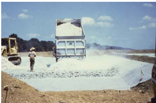
Figure 6.1-26 Aggregate being placed in the infiltration bed
