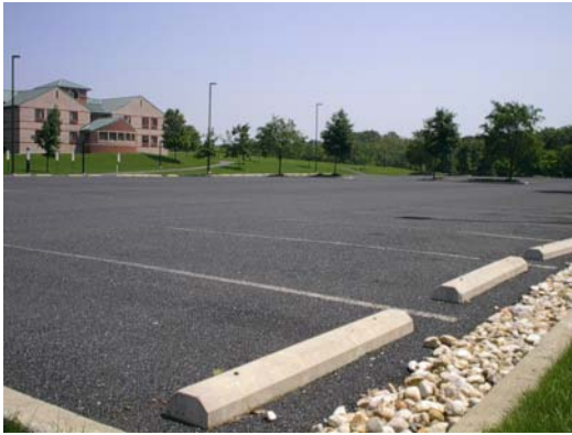
Figure 6.1-12 Porous AC Pavement at Pennsylvania State University, Berks Campus, (CA, 2003)
