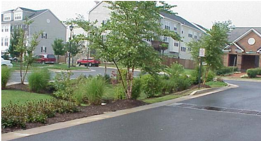
Figure 6.5-4. Trench drain inlet for rain garden in parking lot (LIDC)
