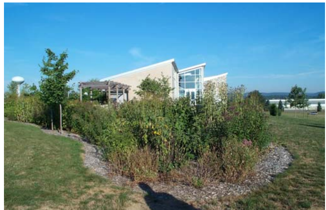
Figure 6.5-16. Rain Garden in State College, PA.
