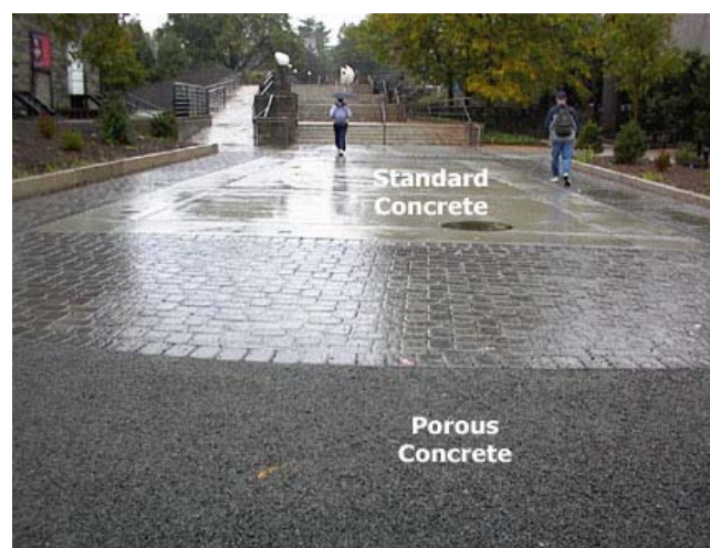
Figure 6.1-8 The edge of this plaza at Villanova University is porous concrete (R. Traver).
