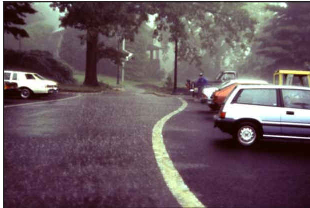
Figure 6.1-1 Porous pavement at the Morris Arboretum, photo taken during Hurricane Floyd, (CA, 1983)
