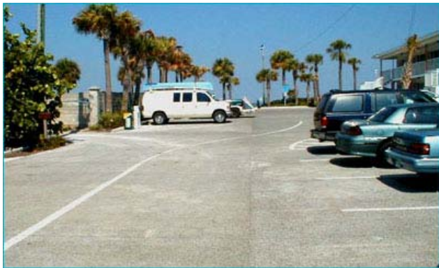
Figure 6.1-6 Porous concrete parking lot ( www.chargerconcrete.com/perviousconcrete.htm )
