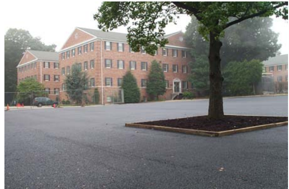
Figure 6.1-13 Porous AC Pavement in Radnor Township, Delaware County (CA, 2003)
