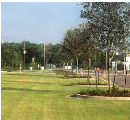
Figure 6.1-10 Seven-acre parking area at Reliant Stadium in Houston, Texas paved with Grasspave. ( www.invisiblestructures.com )
