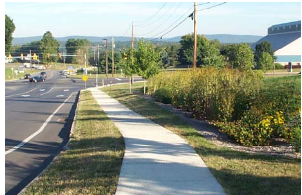
Figure 6.1-15 The Visitor Center at Pennsylvania State University Main Campus used porous concrete to construct the sidewalks, 2000
