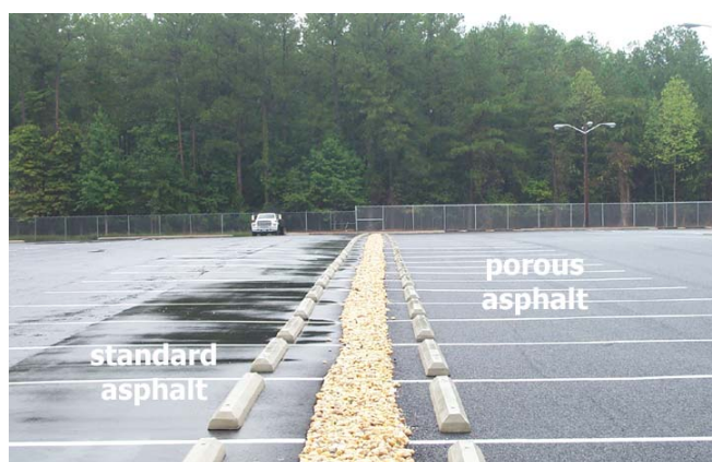
Figure 6.1-3 Standard pavement and porous pavement look very similar
