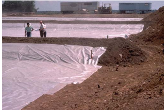
Figure 6.1-25 Unexcavated earthen berms between terraced bed bottoms
