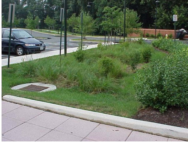
Figure 6.5-6. The surface inlet shown in the lower left provides positive overflow during extreme storm events (LIDC)
