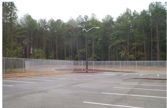
Figure 6.1-7 Porous concrete parking lot at the University of North Carolina, Chapel Hill (CA, 2002)
