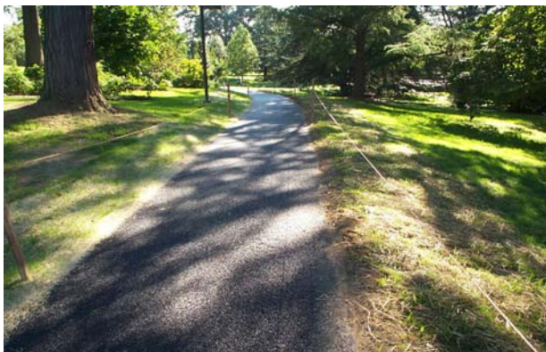
Figure 6.1-14 This pathway at Swarthmore College is made of porous asphalt, with subsurface infiltration bed beneath, 2002
