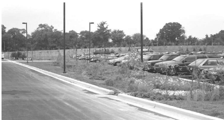
Figure 6.5-13. Curbed parking lot perimeter recharge garden (PGDER, 2002)
