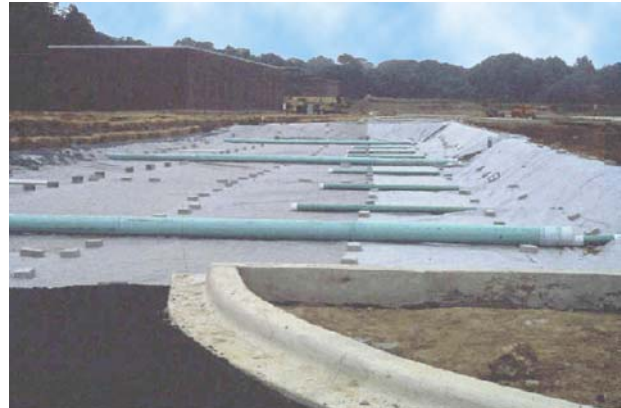
Figure 6.1-18 Roof drains tie directly into the infiltration beds at the DuPont parking lot, (CA, 1985)
