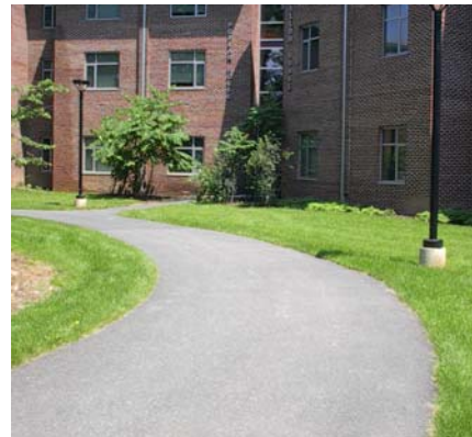
Figure 6.1-11 Standard asphalt pathway with 2ft. reinforced turf edges at Pennsylvania State University, Berks Campus, (CA, 2003)
