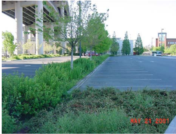
Figure 6.5-12. Parking island rain garden (LIDC)
