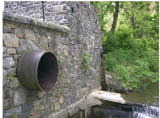
Figure 7-10. Combined Sewer Overflow to the Brandywine Creek (Wilmington, DE).
