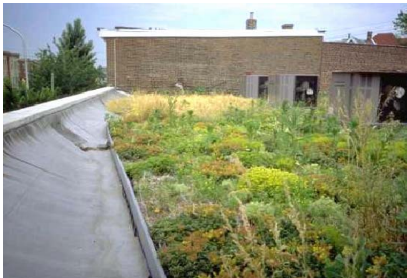
Figure 7-15. Sedum cover on the roof of the Fencing Academy of Philadelphia (Source: Roofscapes Inc.)
