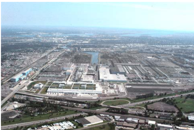
Figure 7-18. Aerial of Ford Rouge Plant.
