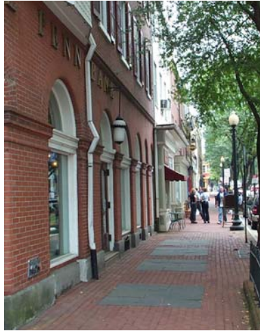
Figure 7-8. Direct connection of roof leaders to storm sewers, West Chester, PA.
