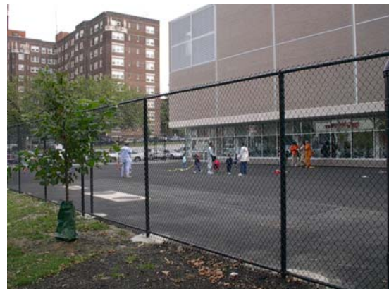
Figure 7-14. Porous asphalt playground w/ subsurface infiltration bed
