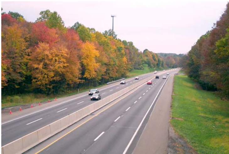
Figure 8-3. Pennsylvania Turnpike (AH)
