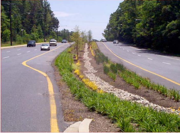
Figure 8-2. Bioretention incorporated in a highway median, (Photo courtesy of LIDC).
