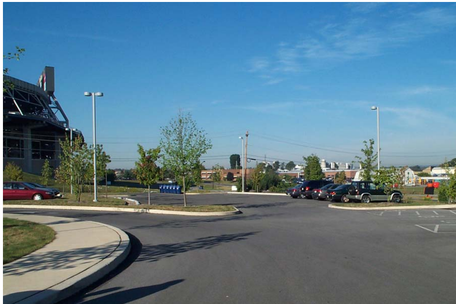
Figure 10-6 Porous asphalt parking lot, State College, Centre County
