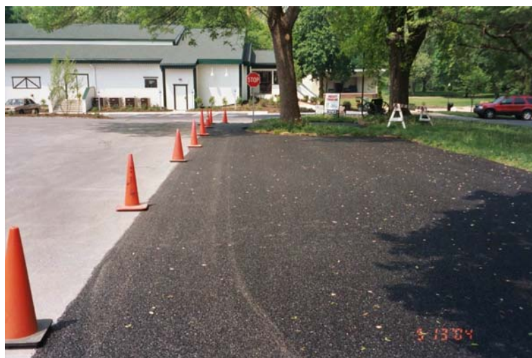
Figure 10-23 Completed porous asphalt parking lot at the Ephrata Performing Arts Center.
