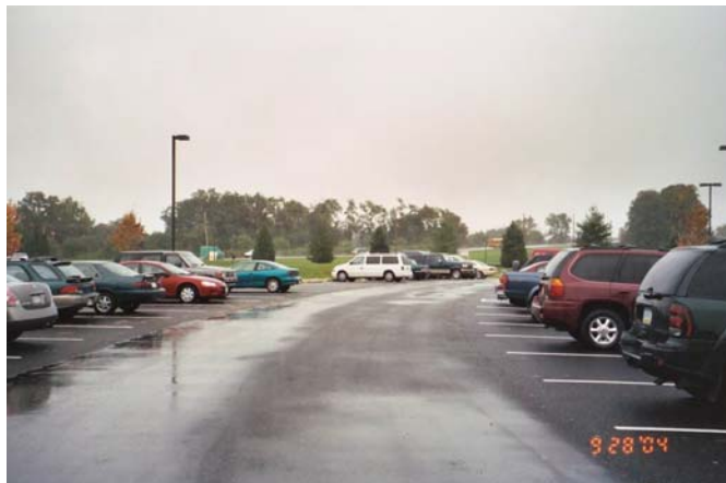
Figure 10-24 Completed porous asphalt parking lot at Lebanon Valley Conservation District
