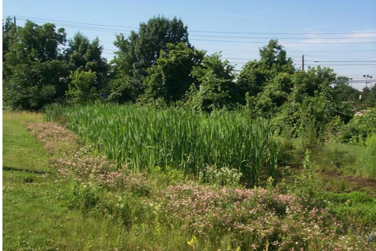
Figure 10-17 Vegetated infiltration filters
