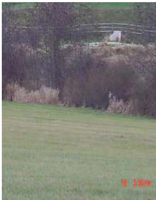
Figure 36. Constructed wetland in background
