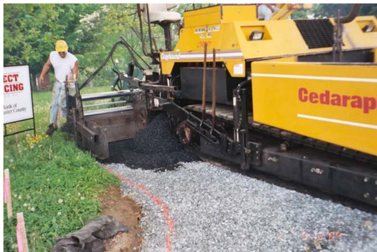
Figure 10-22 Construction of porous asphalt parking area to compliment building expansion.
