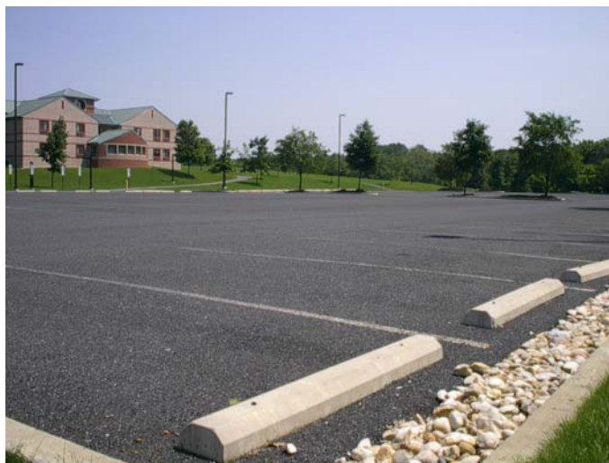
Figure 10-29 Porous asphalt parking lot with subsurface infiltration bed
