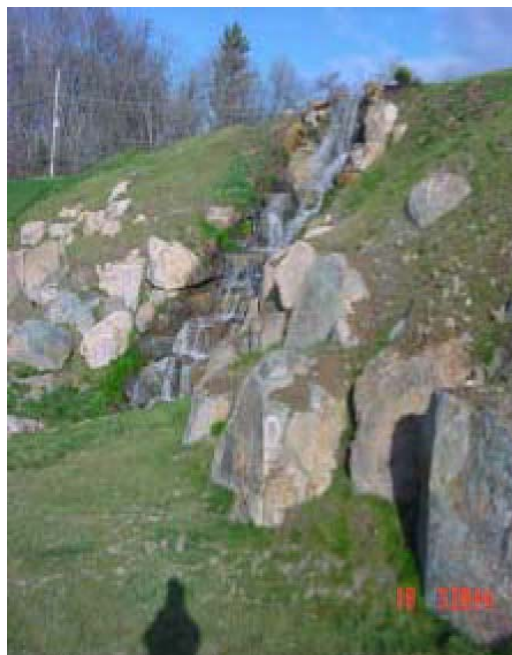
Figure 38. Pond water is pumped up to waterfall and returns to pond through grass swales enhancing aeration
