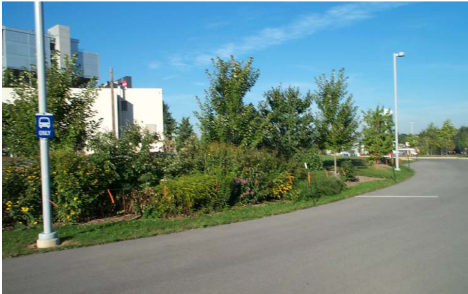
Figure 10-5 Vegetated infiltration bed, State College, Centre County
