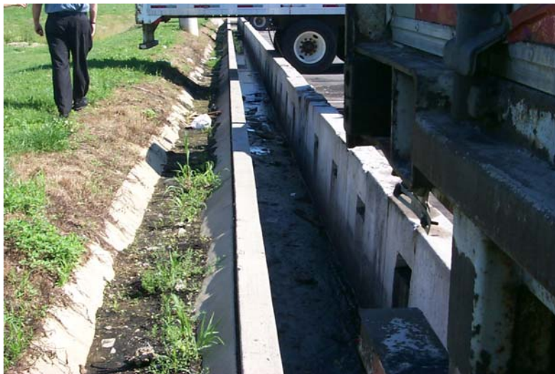
Figure 10-16 Perimeter trench drain
