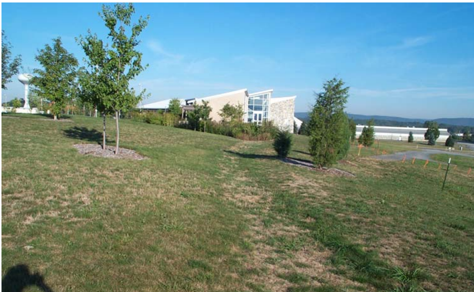
Figure 10-4 Infiltration trench located on contour, State College, Centre County
