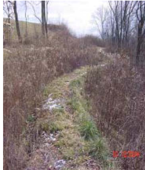
Figure 33. This grassy path is an embankment, or berm, creating depressions for recharge trenches located to the left of the path.
