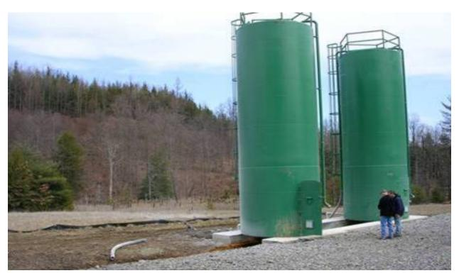
Figure 20. Lime silos for a tipping bucket lime doser treating another mine discharge in the Porcupine Hollow Tributary of Dents Run.
