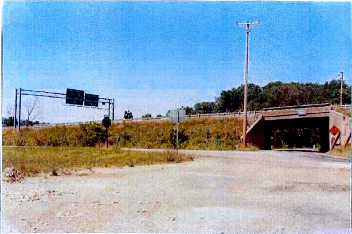
Photo E.1 View looking north at overhead sign (Segment 0220/Offset 1144) and Zediker Station Rd. overpass (Segment 0220/Offset 1370).
