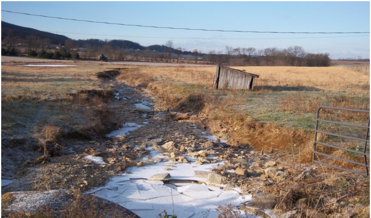
Figure 11. – Active pastureland in-stream, bank destruction, & extensive sediment deposition
