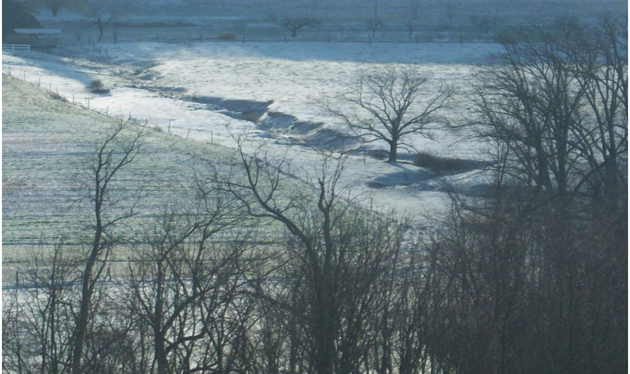
Figure 18. – Headwaters of Dalmatia Run with deteriorating and slumping banks
