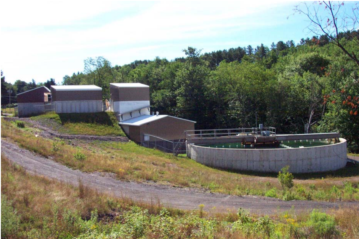
Figure 9. Photograph of the old and new Antrim Treatment Plants, Duncan Township, Tioga County.
