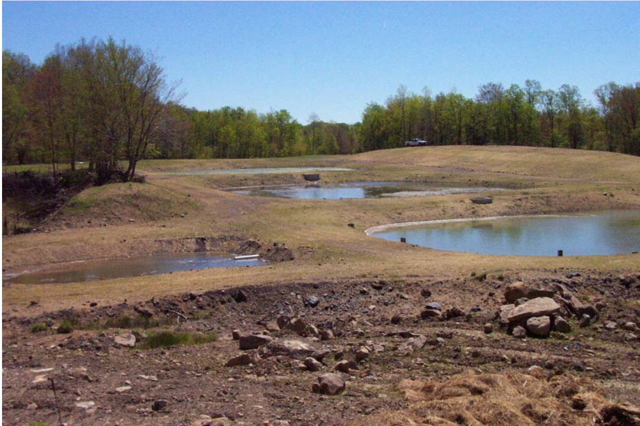
Figure 2. Photograph of the Arnot (State Yard) Treatment System in Bloss Township, Tioga County. The top two ponds are vertical flow ponds that use limestone to generate alkalinity. The pond in the lower right is a settling basin for the precipitation of metal solids and the pond in the lower left is a manganese oxidation pond.
