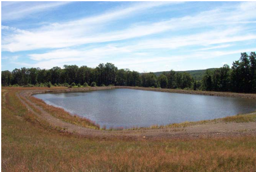
Figure 7. Treatment system at the secondary entry of the Bear Run Mine, Bloss Township, Tioga County.
