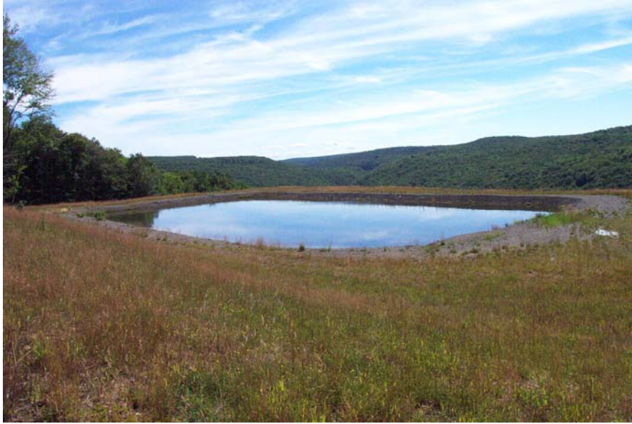
Figure 6. Treatment system at the main entry of the Bear Run Mine, Bloss Township, Tioga County.
