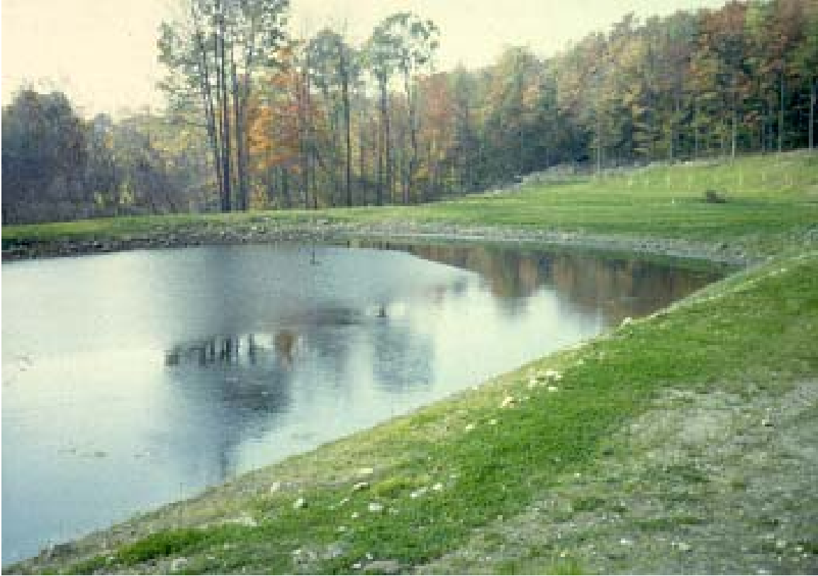
Figure 3. Photograph of the successive alkalinity producing system (SAPS) or vertical flow system near Arnot, Bloss Township, Tioga County.
