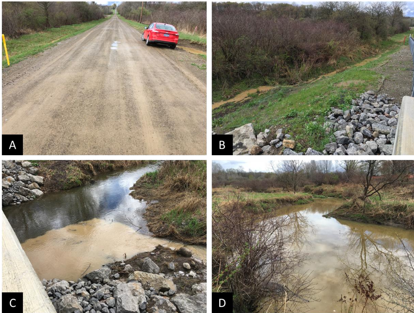
Figure 8. Example of high turbidity caused by an unpaved roads in the Carr Run Subwatershed. Unpaved Road substrate had a large amount of fines (A). Turbid runoff was observed along the road shoulder following a brief storm (B). This created a plume to the stream (C) and high downstream turbidity (D).
