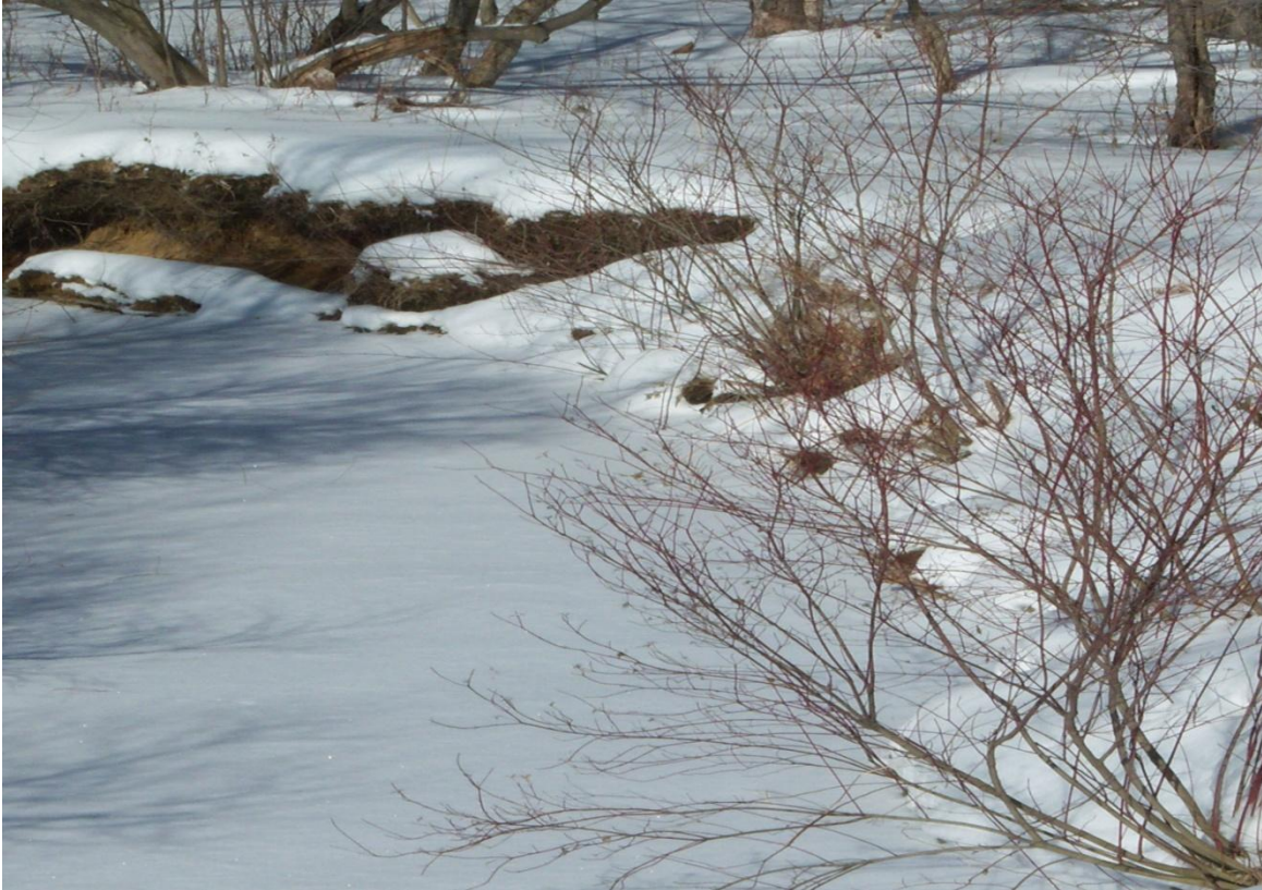
Figure 89. – High prone erosion and slumping banks (with trees) lower section of the headwaters tributary of Chest Creek (looking upstream)
