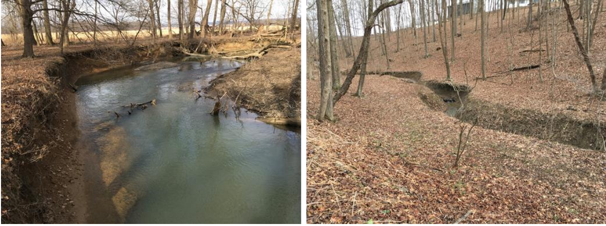
Figure 9. Examples of severe bank erosion in the Chillisquaque Creek Headwaters Watershed.
