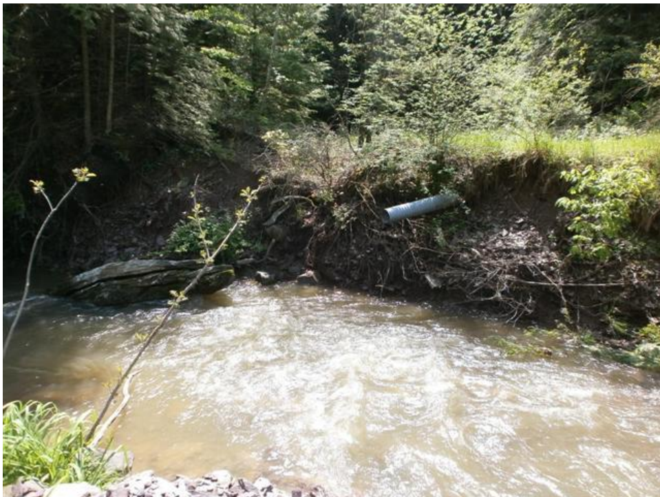
Figure 4. Stream Bank Erosion in the Deerlick Run Watershed
