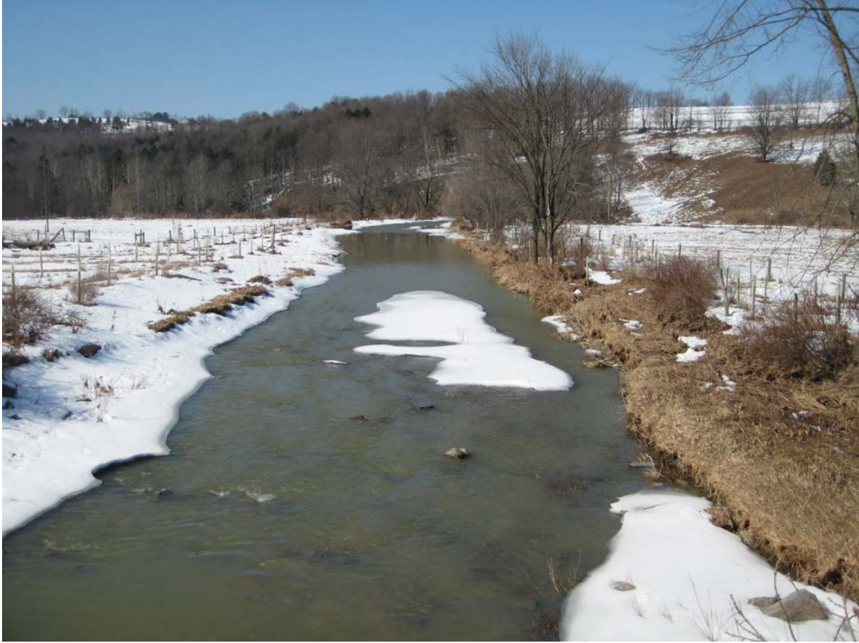
Figure 4. Evidence of Streambank Erosion in the Johnson Creek Watershed (However, the installation of riparian buffers has been completed to help remediate this section of the stream.)
