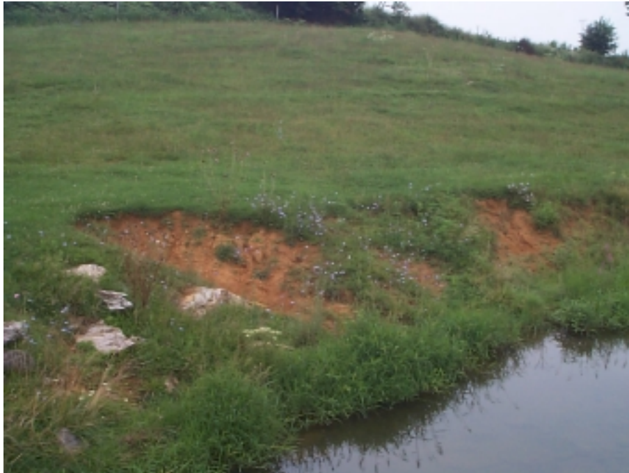
FIGURE 6 - EXAMPLE OF STREAMBANK EROSION IN THE QUITTAPAHILLA CREEK WATERSHED
