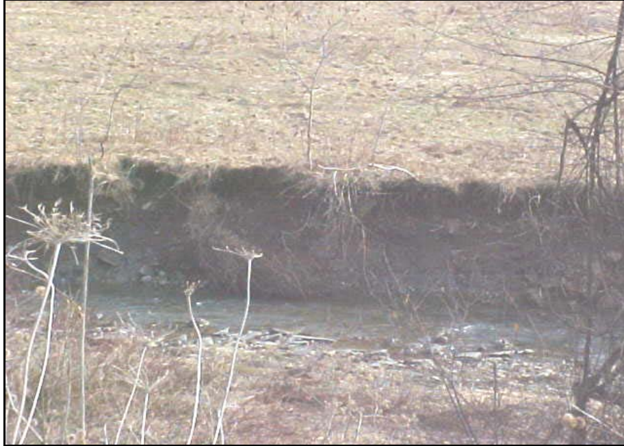
Figure 3. Mainstem UNT French Creek streambank is destabilized.
