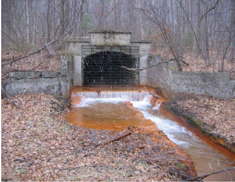
Figure 9. Big Lick Tunnel
