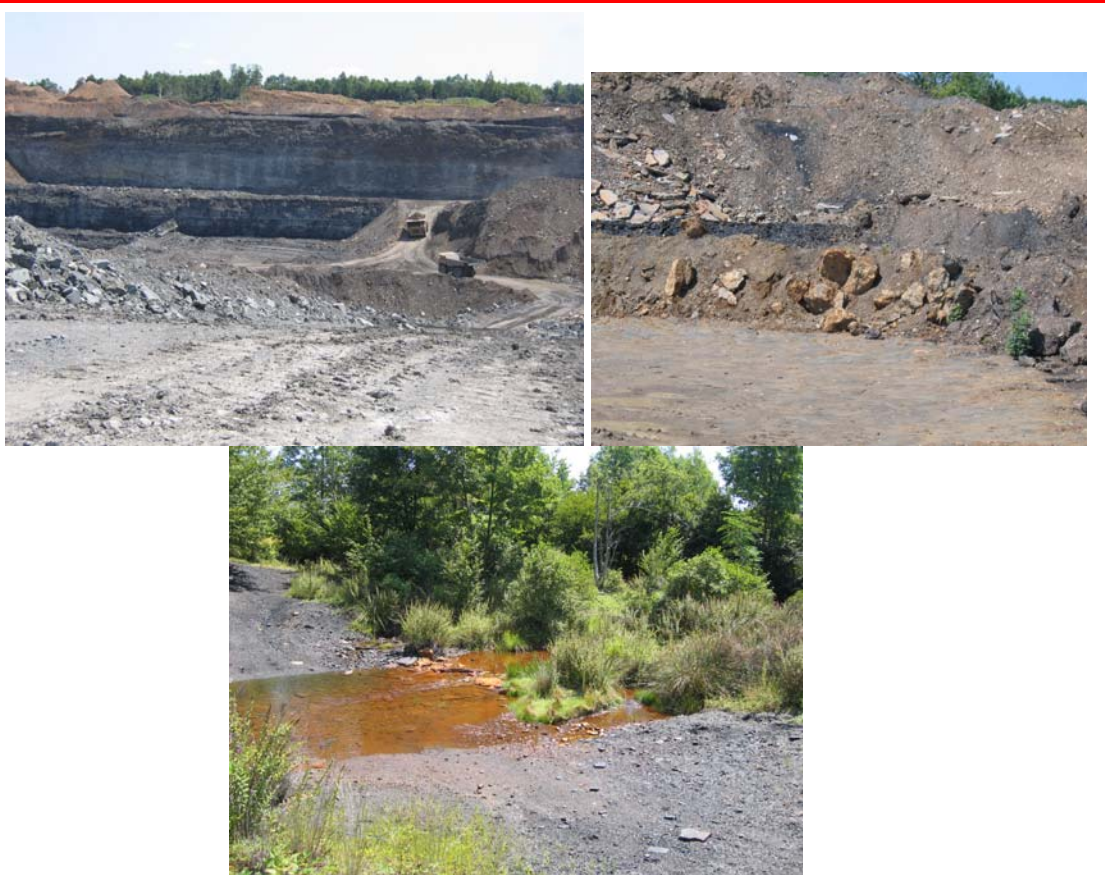
Figure 6. The Kasubic Operation showing the principal pit, and a pit where the Johnstown Limestone is obtained for alkaline redistribution throughout the mine. The lighter colored, irregular-shaped blocks are limestone. XL monitoring point is on Morgan Run, above.
