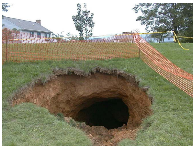
Figure 2-23. New cover collapse sinkhole in a stormwater detention basin in the Ephrata area, Lancaster County, Pennsylvania (Courtesy of William E. Kochanov)
