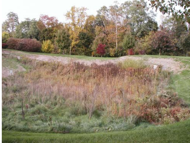
Figure 6.13-5 Constructed Wetland Created from an Existing Detention Basin (Tredyffrin Twp., PA)
