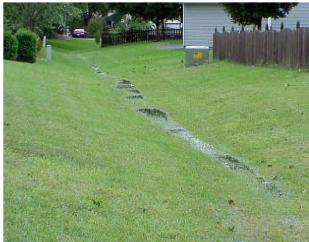
Figure 6.8-5. Vegetated swale along residential area (Virginia Stormwater Management Handbook)
