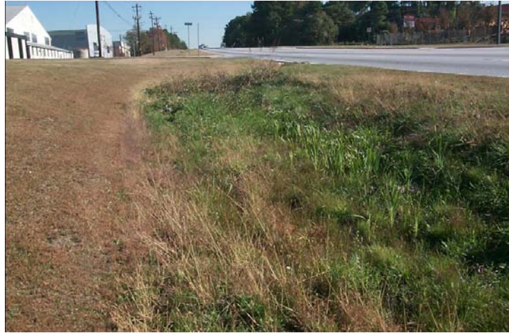
Figure 6.8-6. Vegetated swale along road (Georgia BMP Manual)
