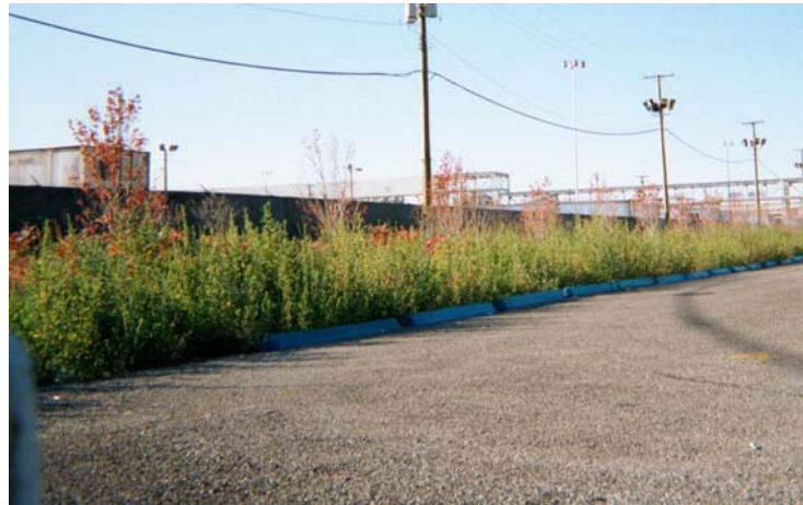
Figure 6.8-2. Vegetated swale along parking area
