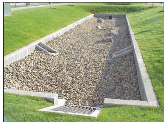
Figure 6.7-4. Contained Filter, (Portland, OR BMP manual)
