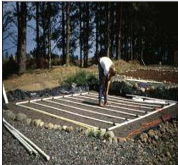
Figure 6.7-8. Laying pipes in a filter. (U of MN, NERC)
