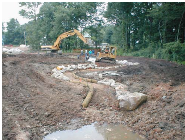
Figure 6.13-6 Example of stabilized inflow channel during construction.
