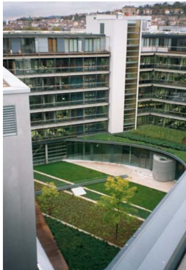
Figure 6.12-3. Vertical storage units for vegetated roof plaza maintenance are common in Germany
