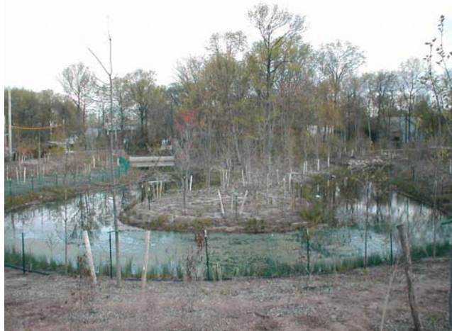
Figure 6.13-7 Example of recently planted constructed wetland.
