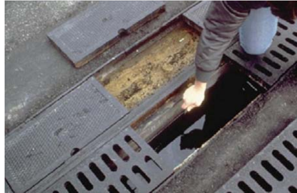
Figure 6.7-5. Perimeter filter (GA manual)
