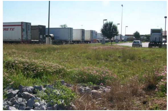
Figure 6.7-2. Vegetated Peat Filter, Carlisle, PA
