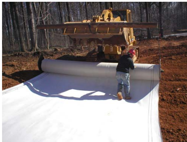
Figure 6.13-8 Installation of Clay Liner
