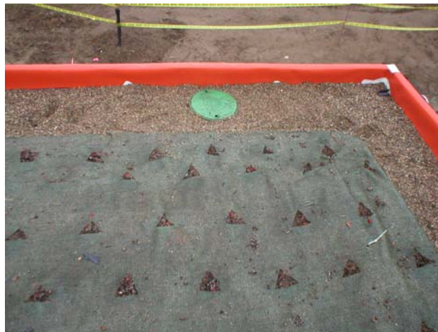
Figure 6.11-2. Stabilization of media during initial planting
