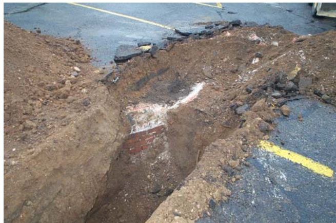
Figure 6.12-7. Excavation of former residential water supply cistern in Ann Arbor, Michigan.
