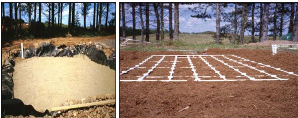
Figure 6.7-1. Surface Sand and Peat Filters (U of MN, NERC)
